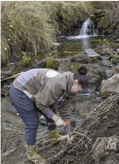
Staking fascines into the stream bank
