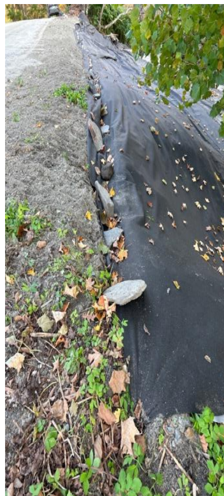
Rocks to help hold fabric at top of TH19 slope
