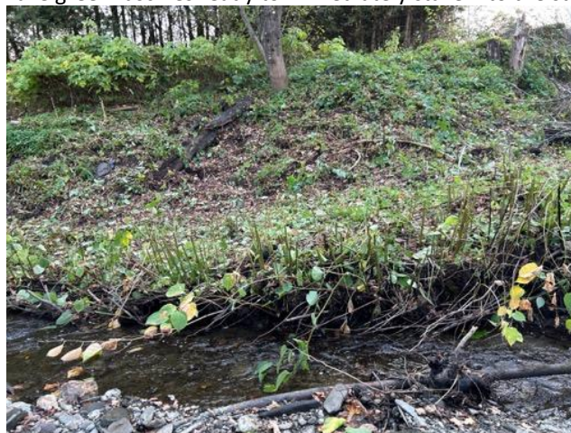
Other students machete-cut JK on the steep slopes alongside Cole Rd where erosion fabric was not installed.
