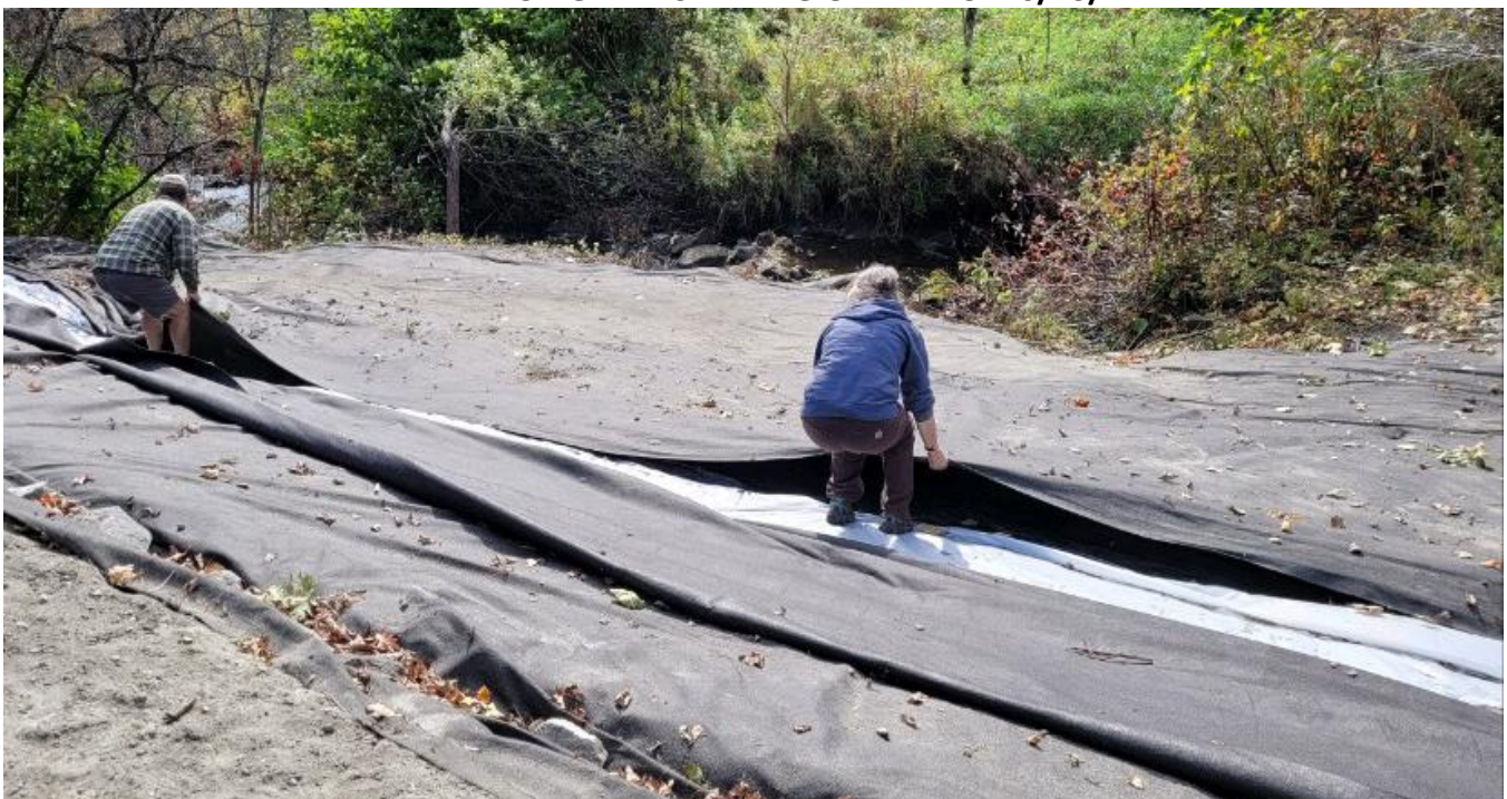
Pulling fabric into place
