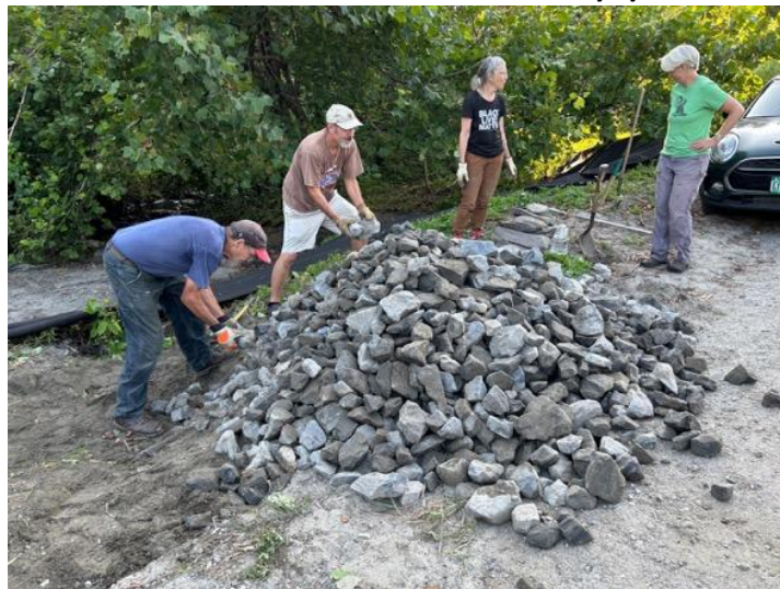
Rocks removed from TH19 gullies for town to take back.
