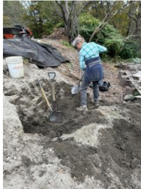
Volunteers dug down 4' to remove JK from the embankment.
